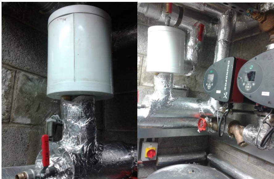
Figure 1 Commercial Tadpole unit 54mm installed.
